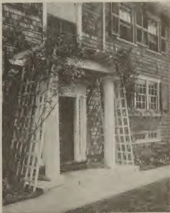
LATTICE USED TO BREAK UP THE FORMAL LINES OF AN ENTRANCE PORCH. SIMPLE, INEXPENSIVE, BUT EXTREMELY EFFECTIVE.
